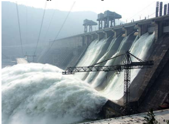
Figure 7.38 Hydroelectric facility (credit: Denis Belevich, Wikimedia Commons)
